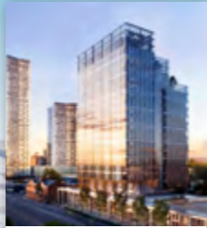
CROWN STREET VICTORIA RESIDENCE Completed
